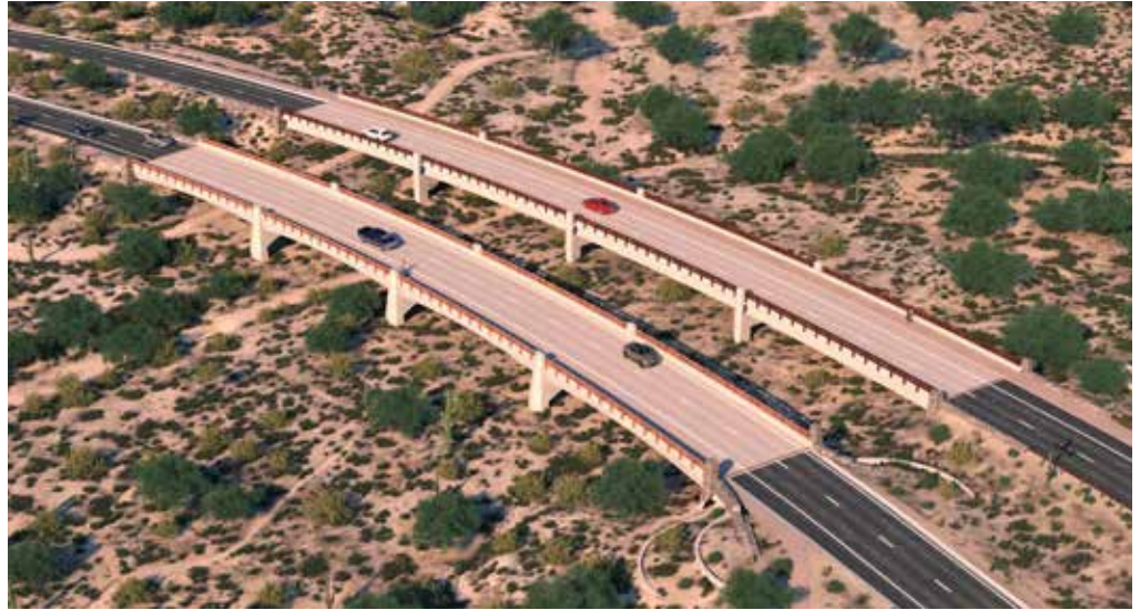
The construction of a westbound bridge on Thompson Peak Parkway over Reata Pass Wash in DC Ranch has been on hold for years.
